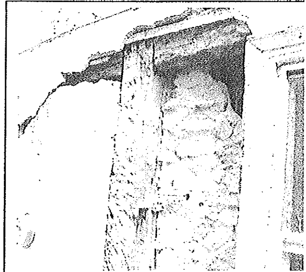
Figure 3. View of exposed frame at the rear building. Note mortise in left post.
