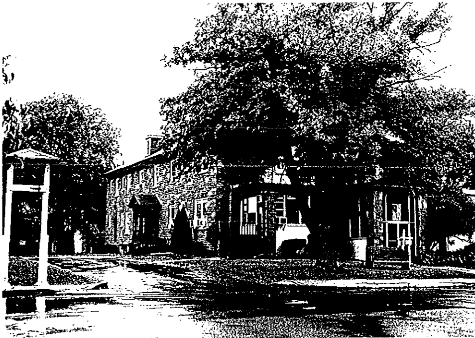
Christ's Home for Children: Photo 3— Looking southwest towards the front and southeast façades of the administration building.
