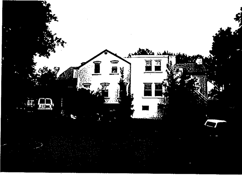
Christ's Home for Children: Photo 24 — Looking southwest towards the rear façade of the “Senior Boys” residence.
