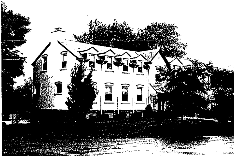
Christ's Home for Children: Photo 23 — Looking northeast towards the front and west façades of the "Senior Boys" residence.
