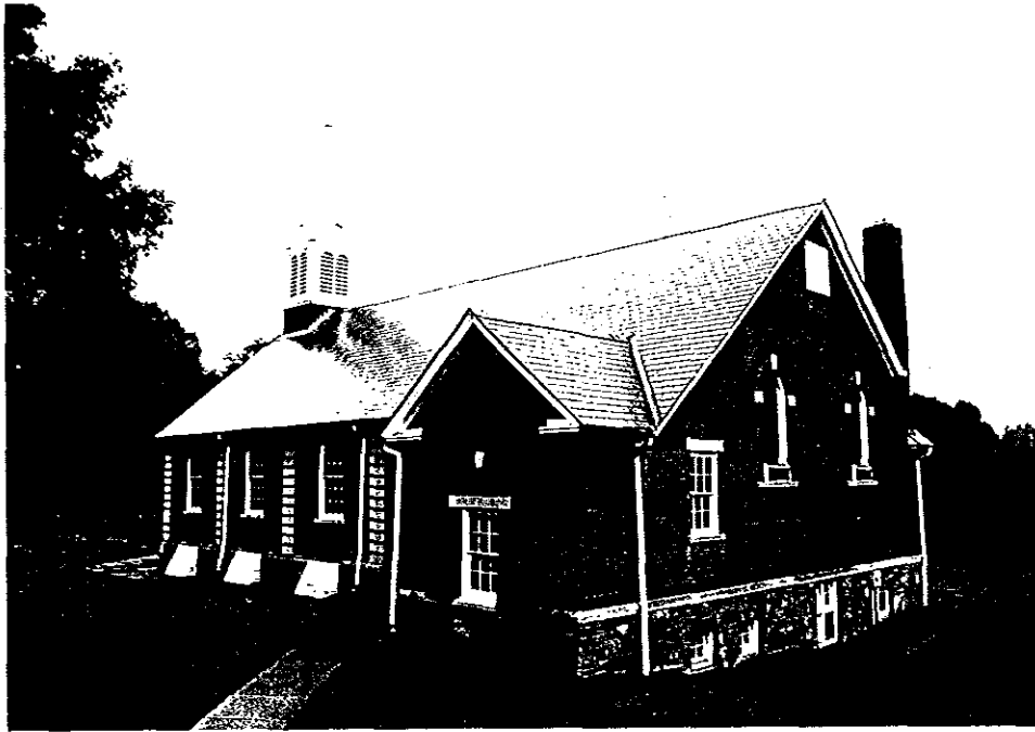
Christ's Home for Children: Photo 2 — Looking east towards the rear and north sides of the chapel.
