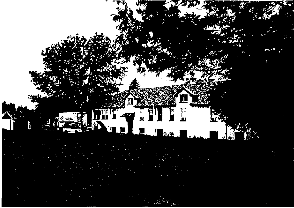
Christ's Home for Children: Photo 20 — Looking northwest towards the rear and east façades of the "Senior Girls" residence.
