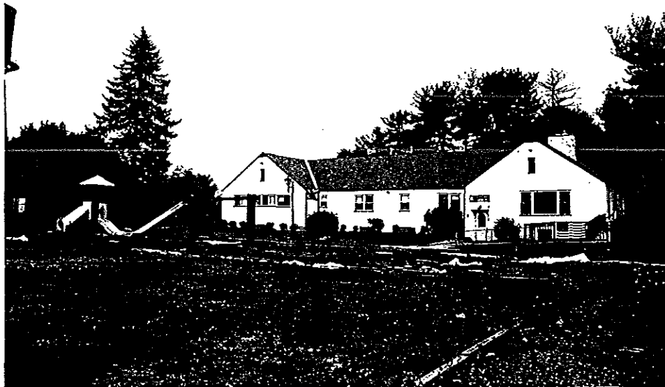
Christ's Home for Children: Photo 13 — Looking southeast towards the front and west sides of the "Intermediate Boys" residence.
