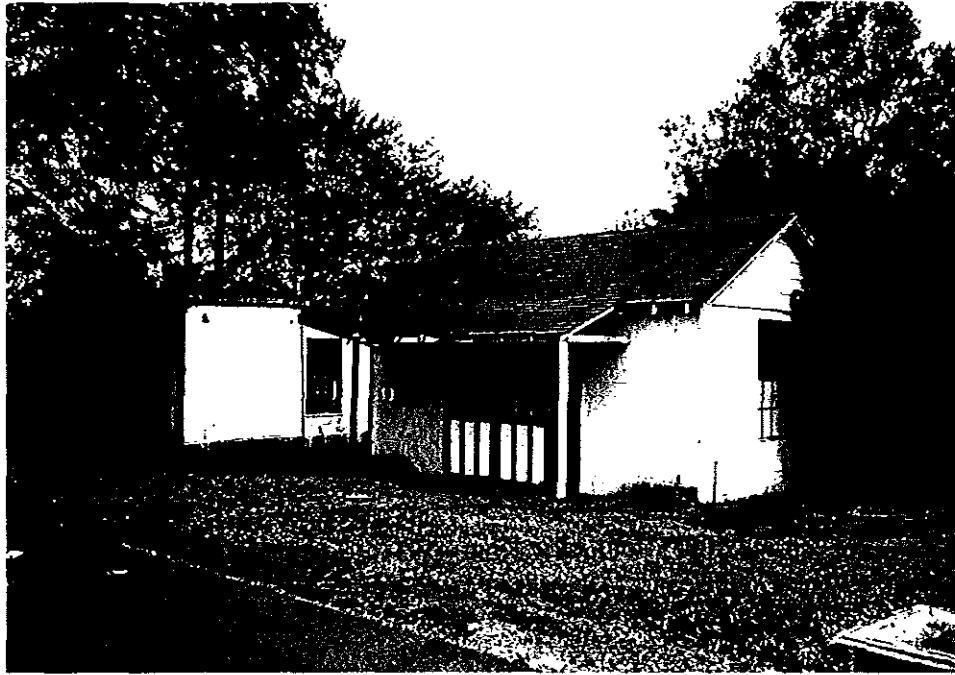
Christ's Home for Children: Photo 6 — Looking southeast towards two utility buildings, an electrical building and a garage.
