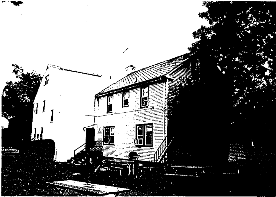
Christ's Home for Children: Photo 8 — Looking northeast towards the rear and northwest façades of the "Primary Boys" residence.
