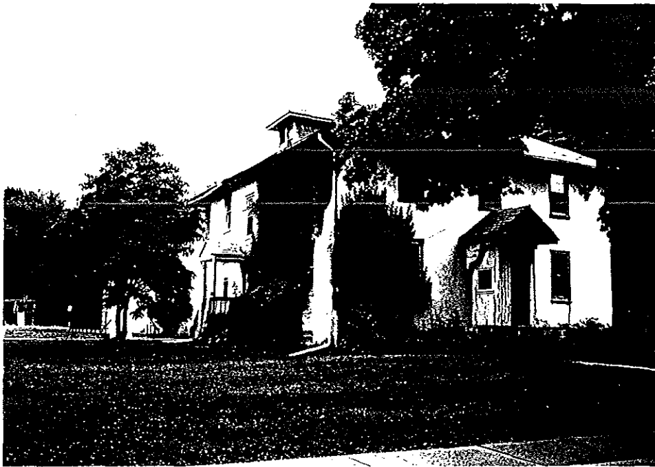
Christ's Home for Children: Photo 17 — Looking southwest towards the front and east sides of the “Junior and Intermediate Girls” residence.
